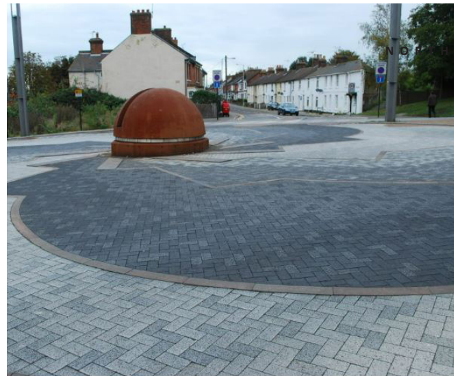
Shared surface treatment
