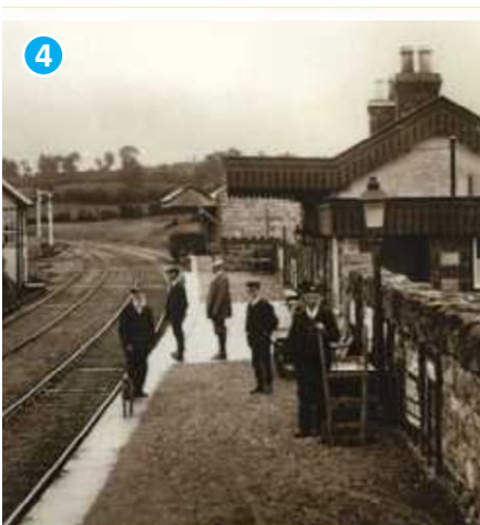
Source: Historical Picture Archive
