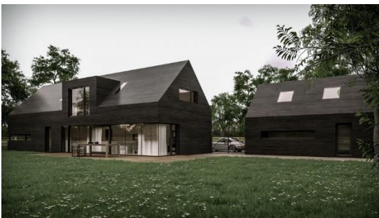
Fig. 13.22 – The massing of the building forms are appropriately relaxed by the positioning of the window on the corner. The extended dormer window at first floor also has the same fenestration from ground floor carried up which break up the extent of roof at first floor. (Patrick Bradley Architects)
