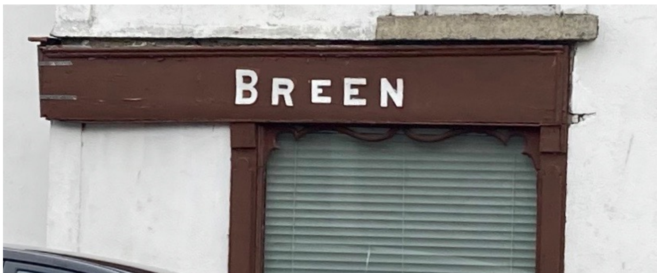
Cusped foils in corners and scrollwork detail along head
