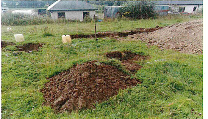
TEST HOLES AS DUG ON SITE.
