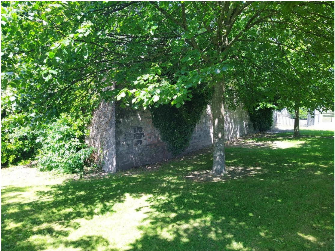
Figure 18: Rear, east, wall of former courthouse building marked on first edition Ordnance Survey map, forming west boundary of the proposed development area, from south-east.
