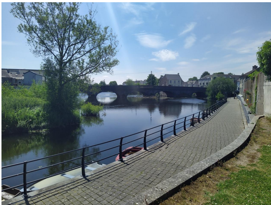
Figure 14: Graiguecullen bridge from west.
