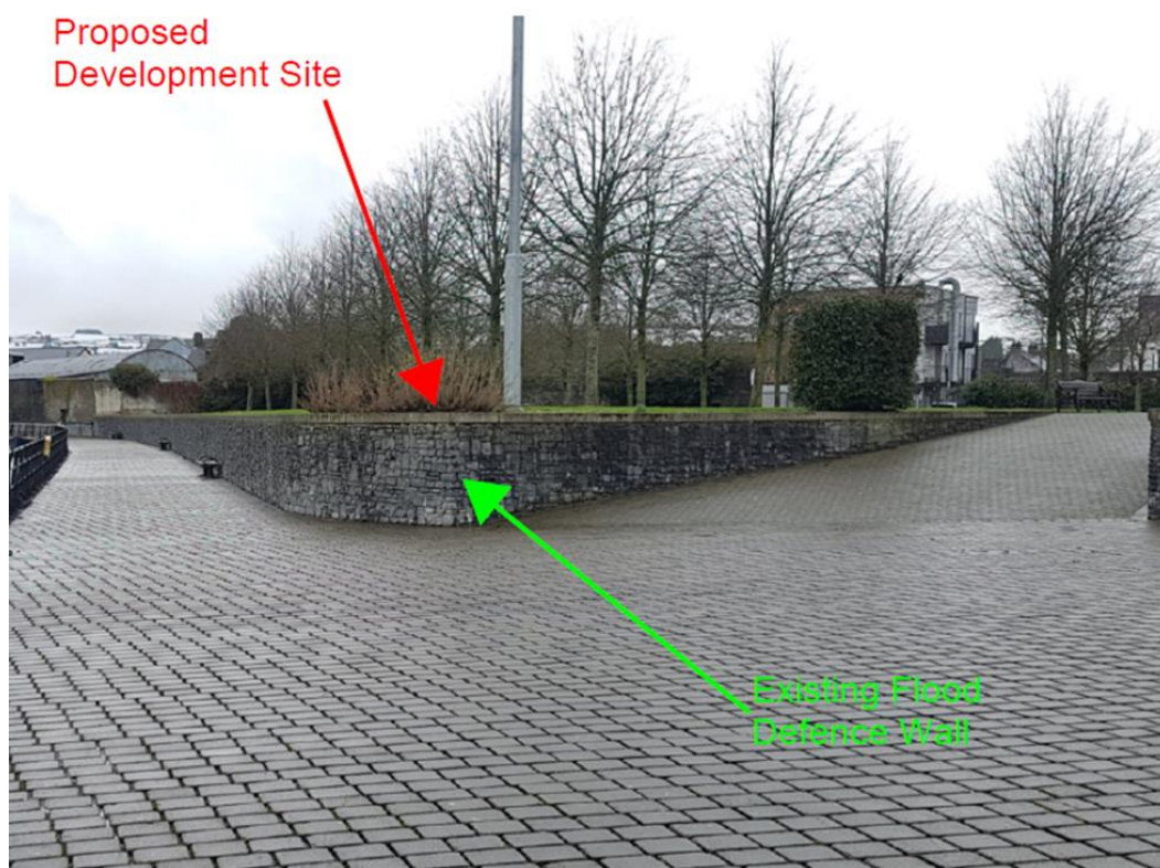
Figure 2 - Existing Flood Defence at 'Site A'
