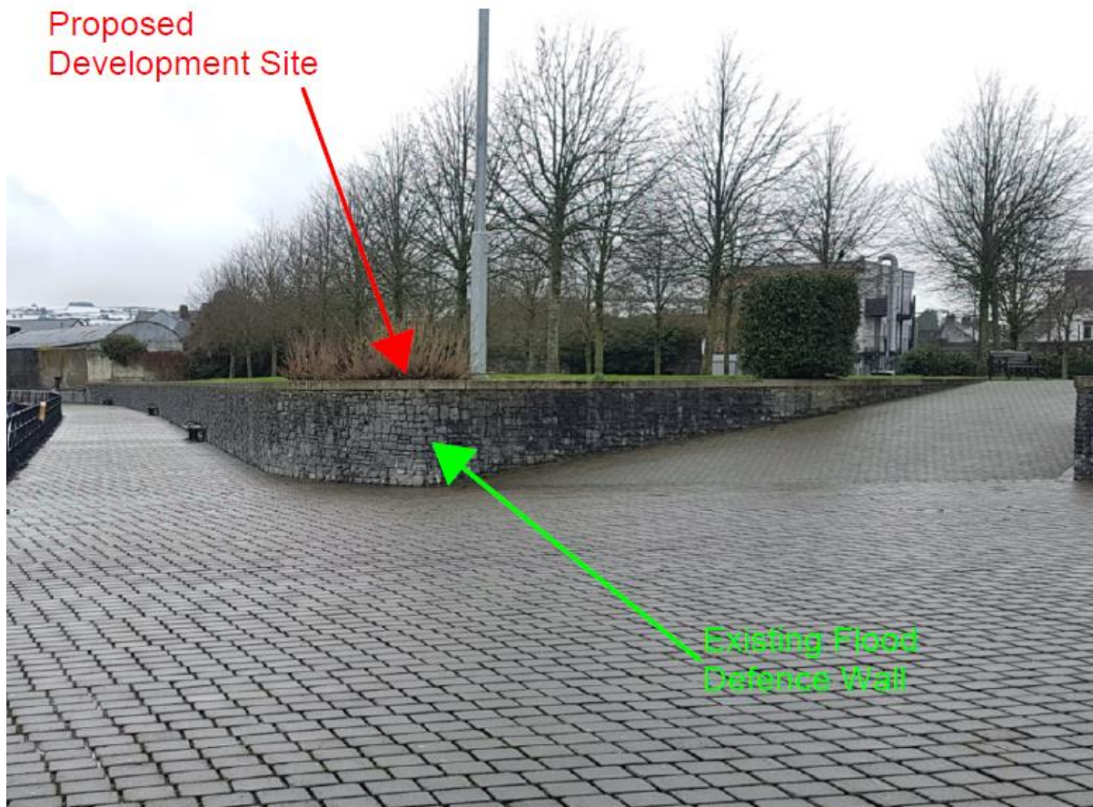
Figure 2 – Existing Flood Defence at 'Site A'
