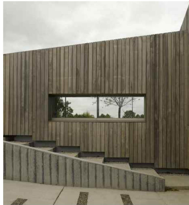
Thermally modified cladding on 'Old Bearhurst'
