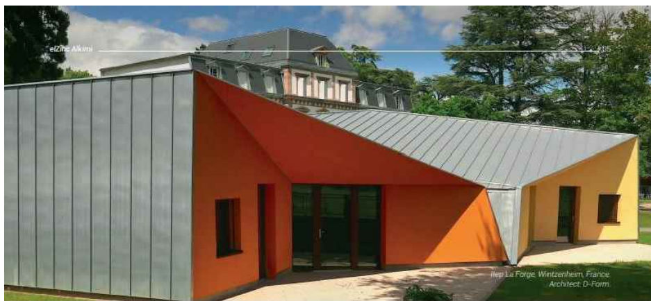
Titanium finish to elZinc standing seam cladding
