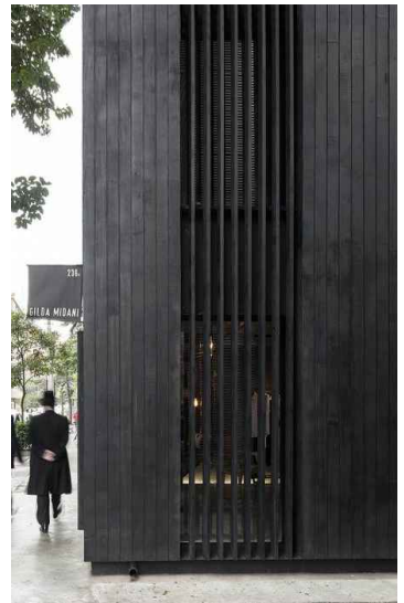
Timber rainscreen in front of window
