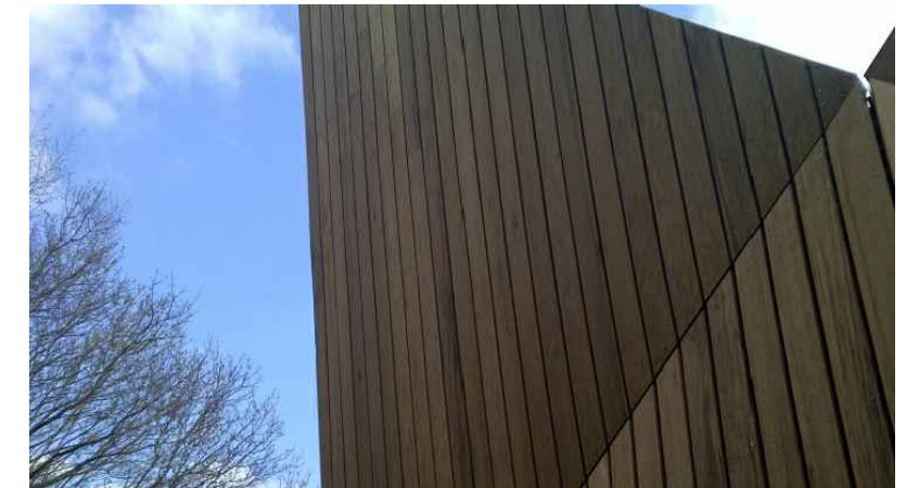
Thermally modified cladding on swimming pool in Beaconsfield London 2
