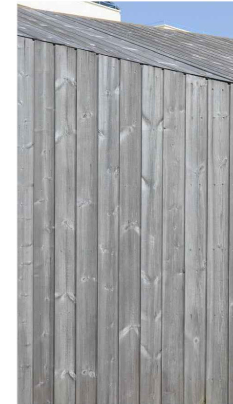
Even weathering of cladding as indicated
