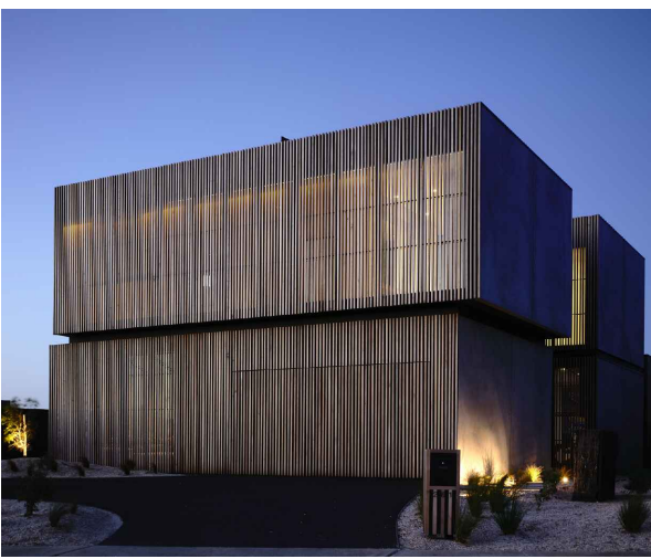
Torquay House, Australia - rainscreen cladding
