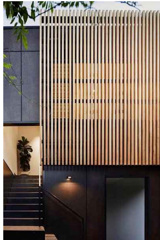
Dark cladding in conjunction with timber rainscreen
