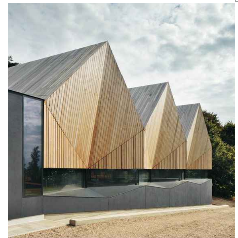
Thermally modified cladding on swimming pool in Beaconsfield London 2
