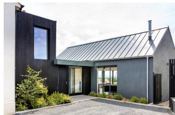
Fig. 13.42 –Well defined forms are used with a clear hierarchical relationship to the existing dwelling. (Cairnview House Extension by BGA Architects)
