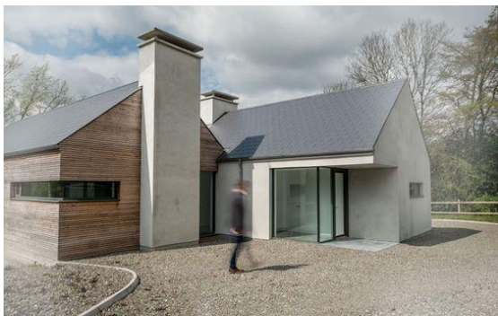
Fig. 13.18 –The proportions and expression of the chimney breast are a clever reinterpretation of the traditional forms. They offset and contrast well with the material palette used. The proportions of the glazing balance the contrasting materials used. (Simply Architecture)
