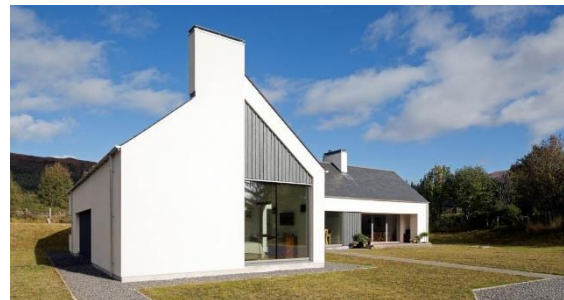
Fig. 13.12 – Simple forms are used to reflect typical rural cottage vernacular with a contemporary interpretation and to a higher standard such as this passive house example. (Tigh na Croit by HLM Architects)
