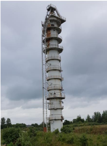
Figure 1: Former Lime Kiln Cooling Tower
