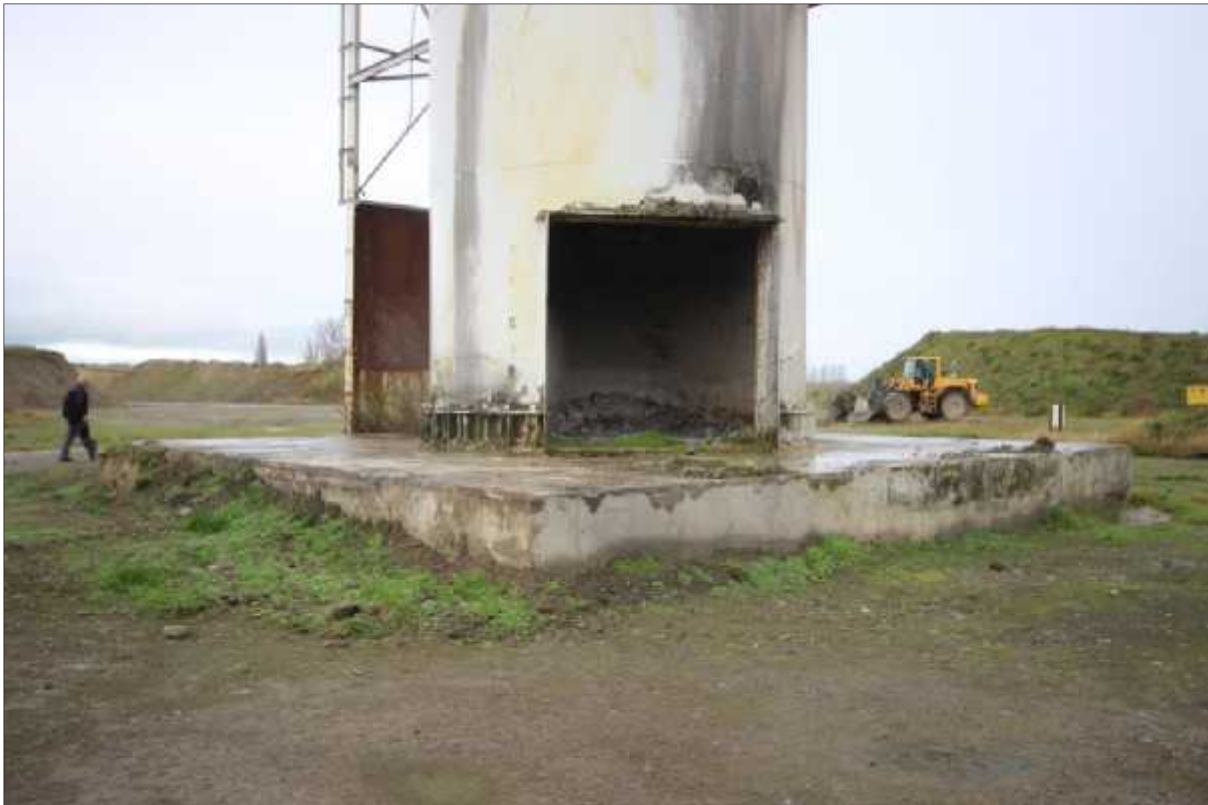
Plate 3: Reinforced concrete base to the lime kiln
