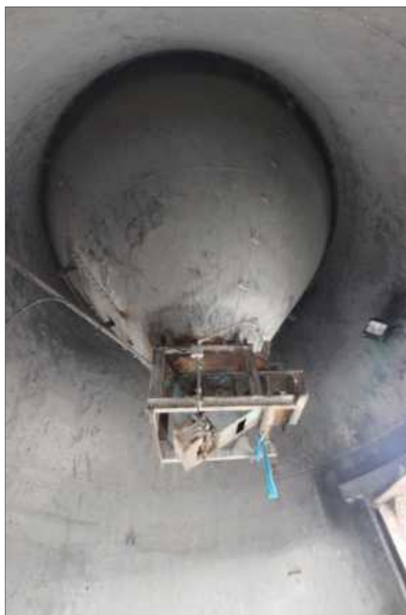
Plate 4: Base of the kiln (within the tower base)
