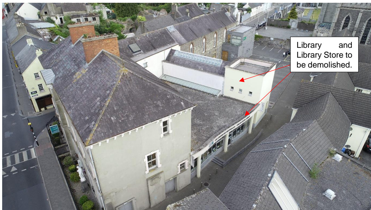
Figure 6 Proposed Building to be demolished
