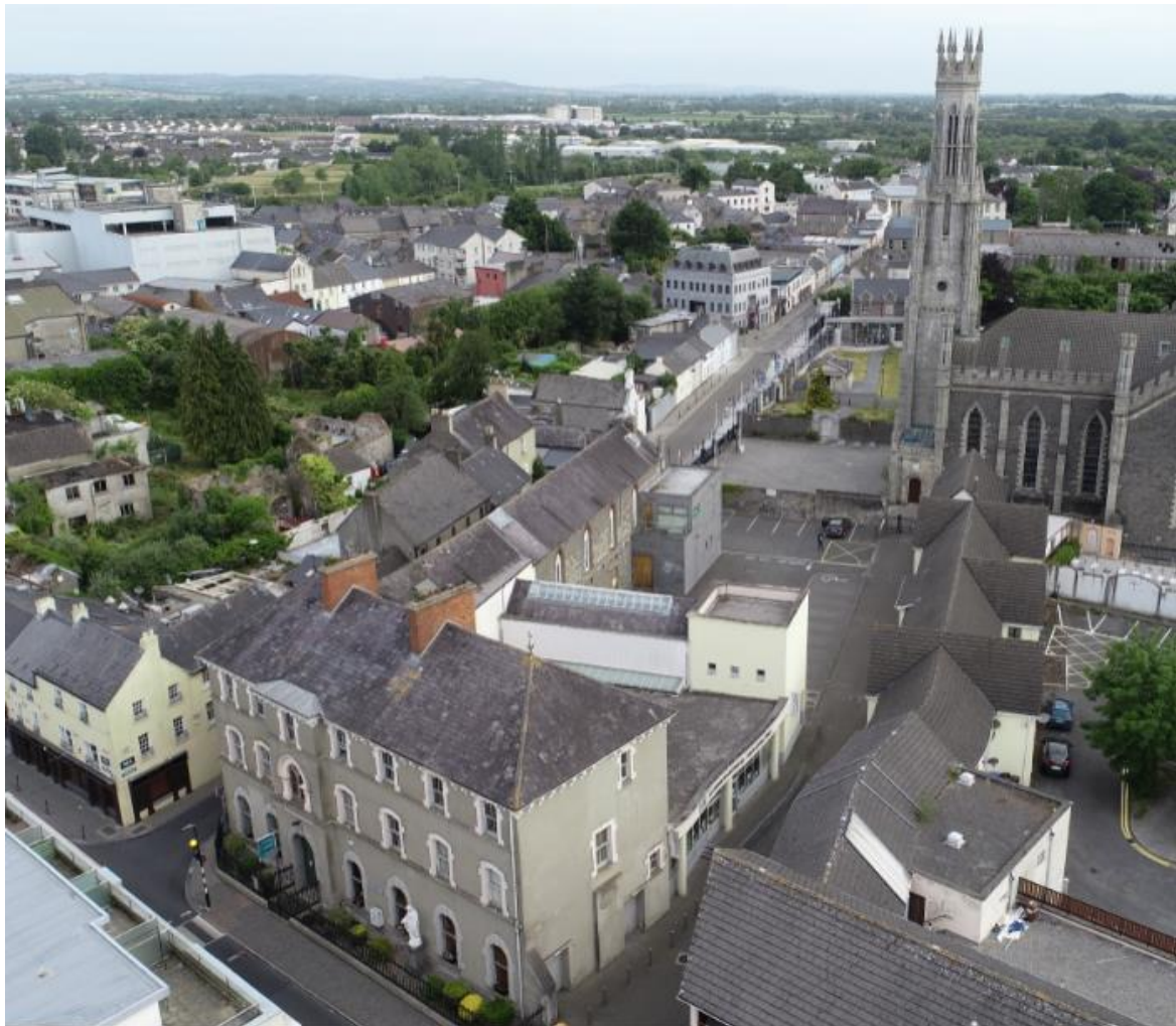
Figure 6 Aerial Image of Site
