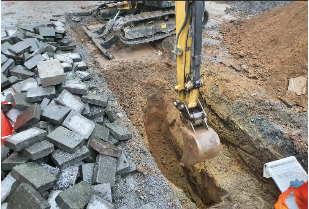
Plate 13 - Geotechnical Test Pit 2, looking southwest
