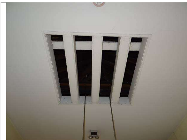
Fig.48: Rods installed to suspend staircase.
