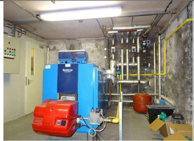
Fig.96: Basement, west bowed room, looking east
