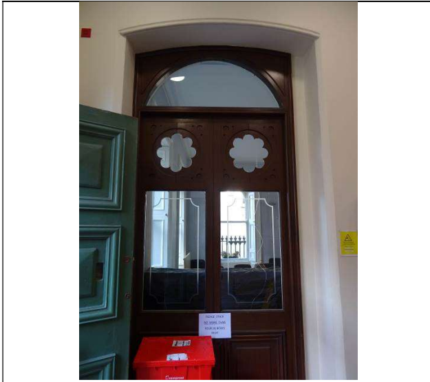
Fig.105: Main entrance hall, window to Shaw Room
