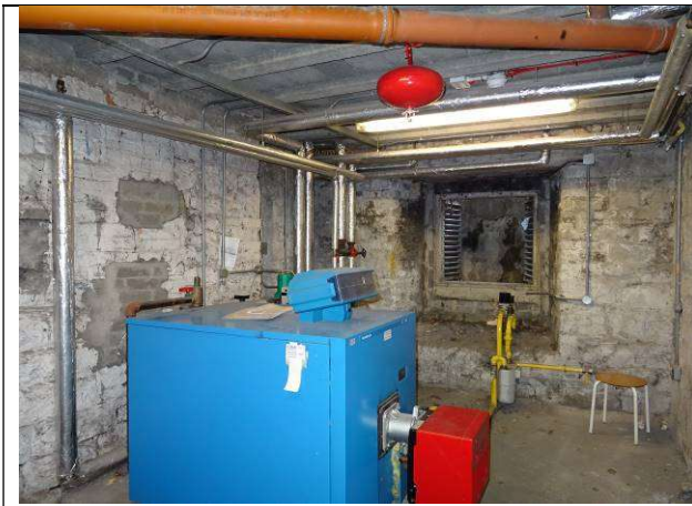
Fig.89: Basement, west room, looking south
