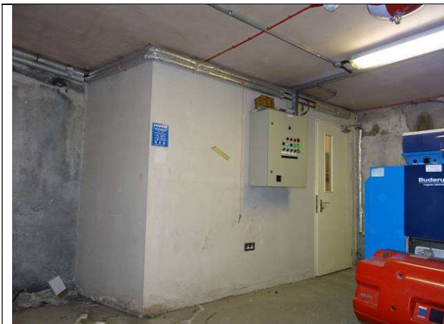
Fig.97: Basement, west bowed room, looking south
