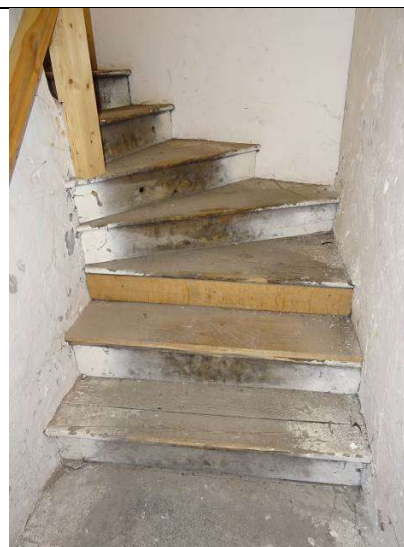
Fig.88: Stairs descending to basement
