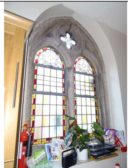
Fig.180: First floor, kitchen ledged lights
