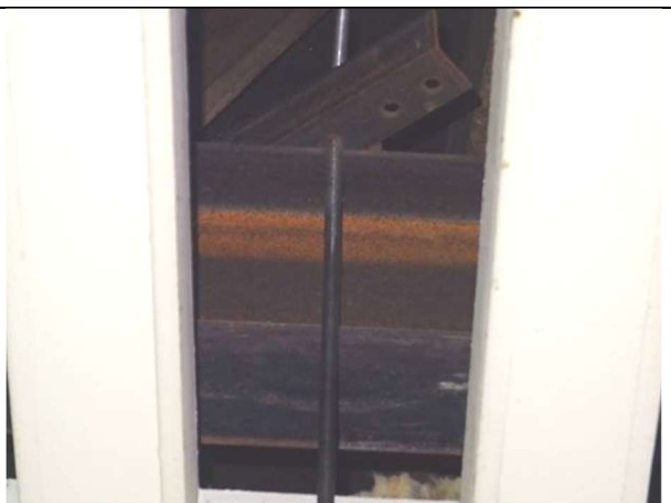
Fig.49: Rods are suspended from attic level.
