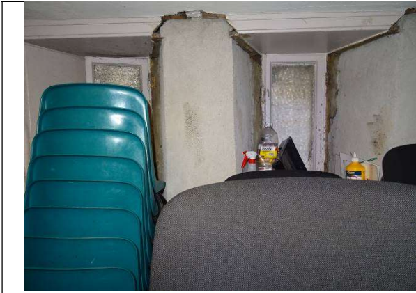
Fig.141: Windows to west room behind stairs
