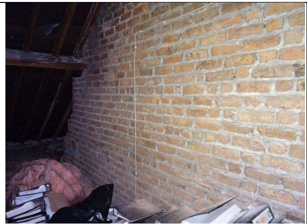
Fig.198: Eastern red brick chimneystack
