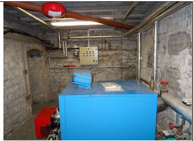
Fig.90: Basement, west room, looking north
