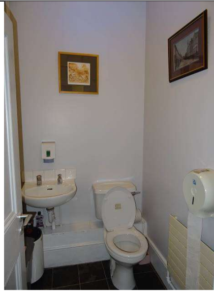
Fig.172: One of two WCs to first floor hallway
