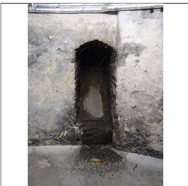
Fig.99: Coal hole chute to west bow in basement
