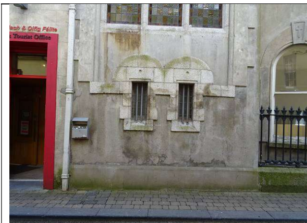
Fig.81: Ground-floor of stairs bay to west
