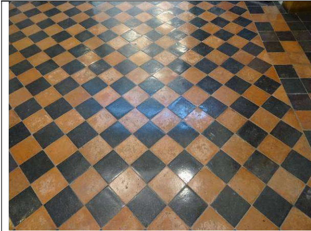
Fig.44: Shellac-coated quarry tiles to stairhall floor.
