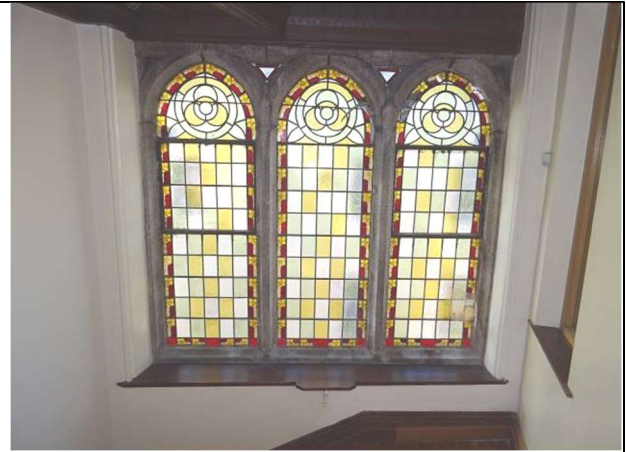
Fig.148: Leaded lights at first half-landing
