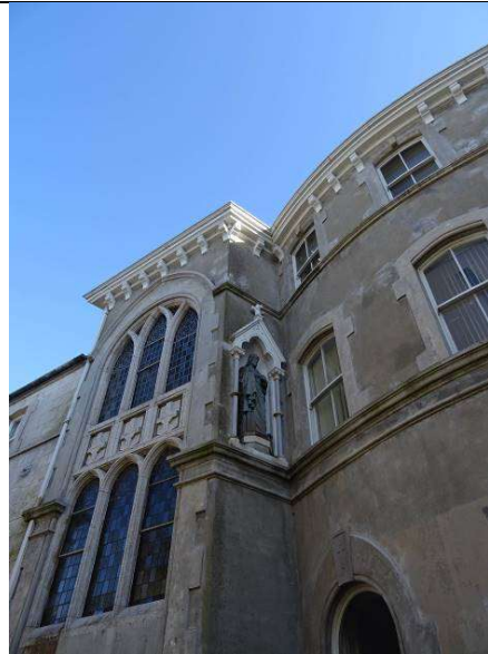
Fig.84: Niche and leaded lights windows to west
