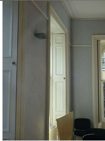
Fig.112: Flat-pannelled shutter to front elevation
