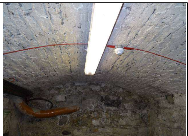
Fig.94: Basement, mid room, vaulted ceiling
