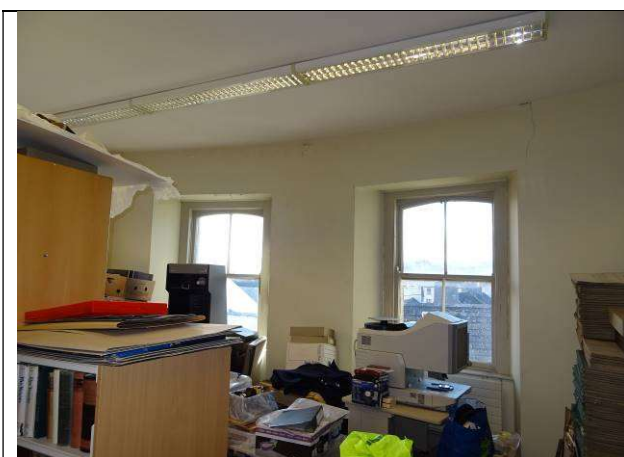
Fig.187: Second floor, archive, bow-ended room to west, looking west
