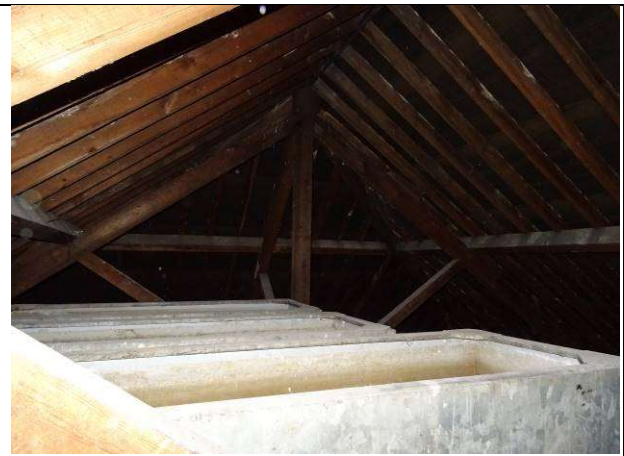
Fig.196: Three open water tanks to east end of roof
