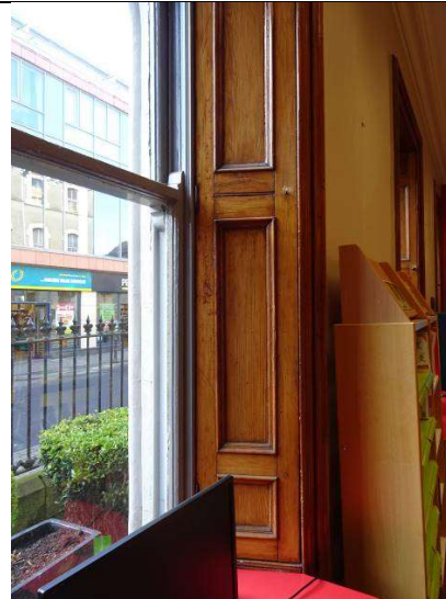
Fig.136: Detail of flat-panelled shutter to window on front elevation of children's reading room
