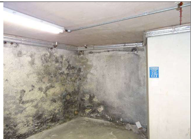
Fig.98: Basement, west bowed room, looking NW
