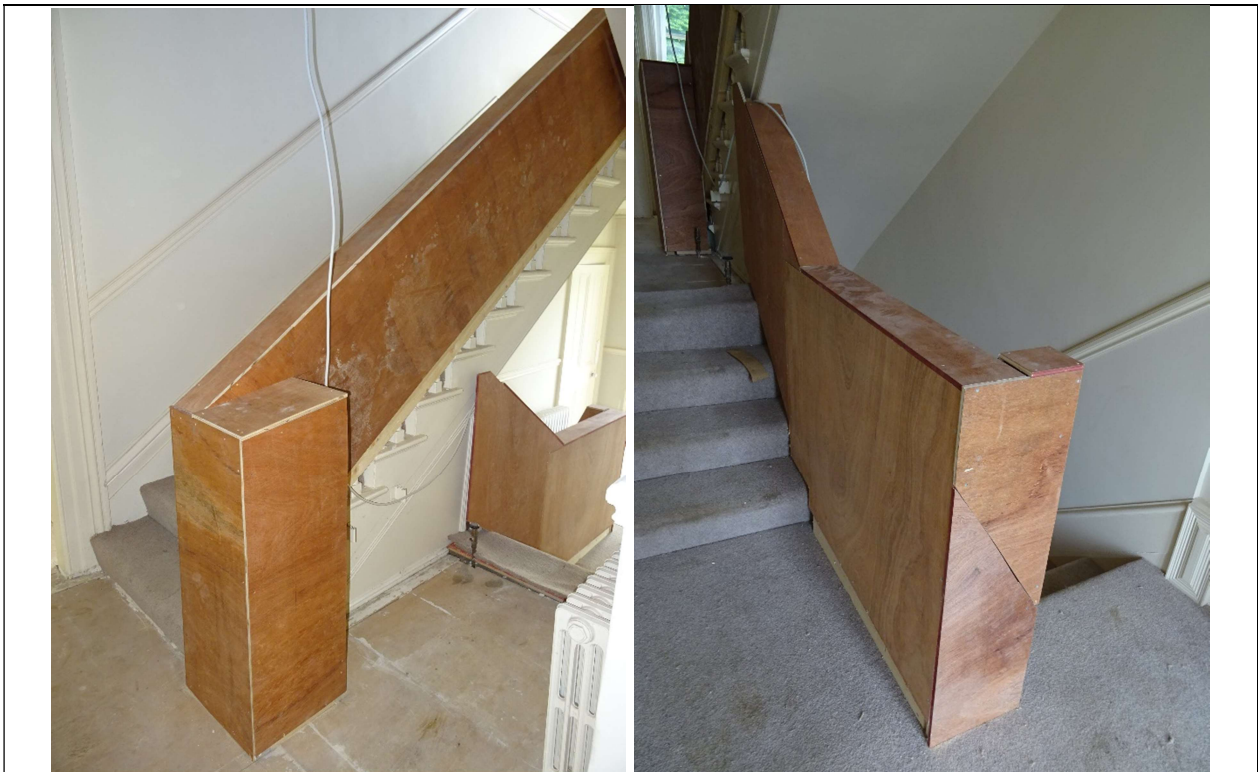
Fig.62: Images of staircase protected by means of plywood sheeting during works.
