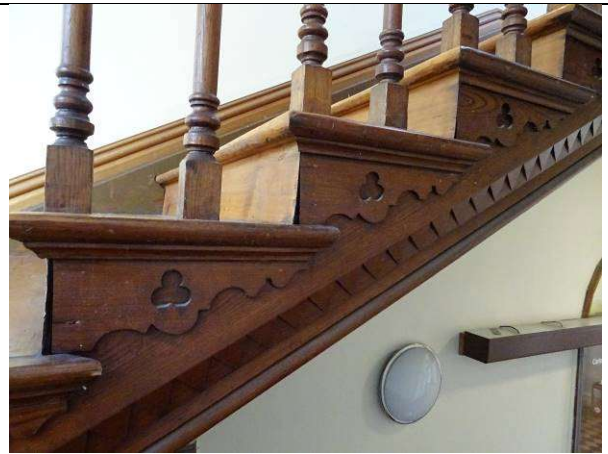
Fig.47: Treads of stairs projecting forward.
