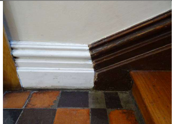
Fig.118: Stucco skirting board and timber wall string at foot of staircase
