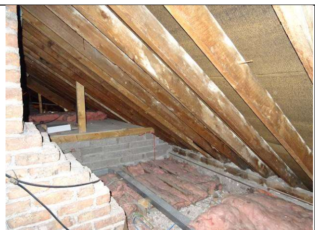
Fig.200: Concrete blockwork to top of lift shaft
