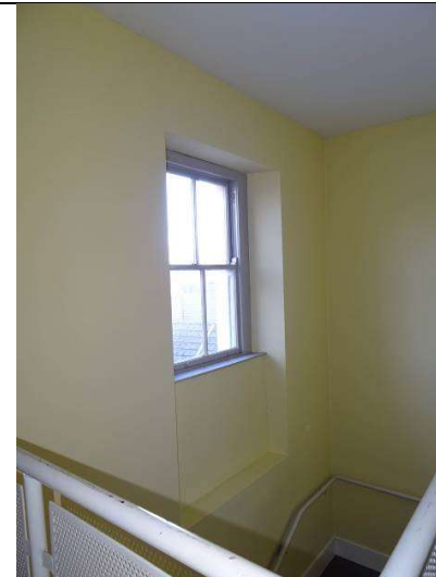
Fig.162: Second-floor window at Window to north wall at second floor
