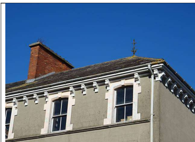
Fig.69: Hipped slate roof over east end of building
