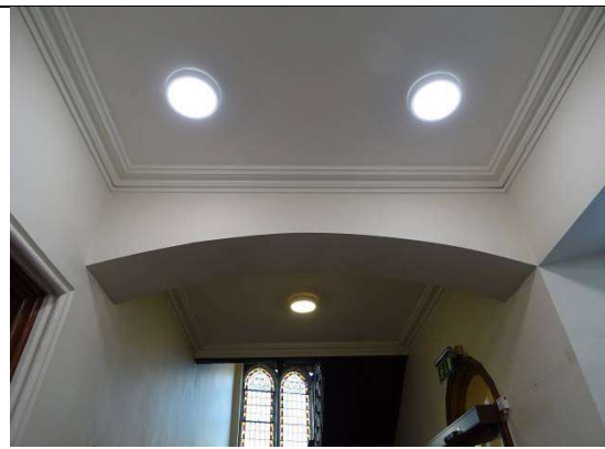
Fig.114: Archway and ceiling to stairhall
