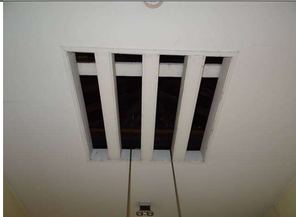
Fig.155: Opening to roof space through which staircase suspension rods hang
