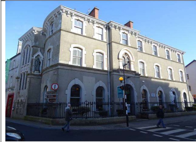
Fig.65: South-facing front elevation
