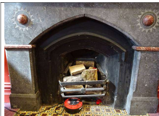
Fig.133: Cast-iron fire grate
