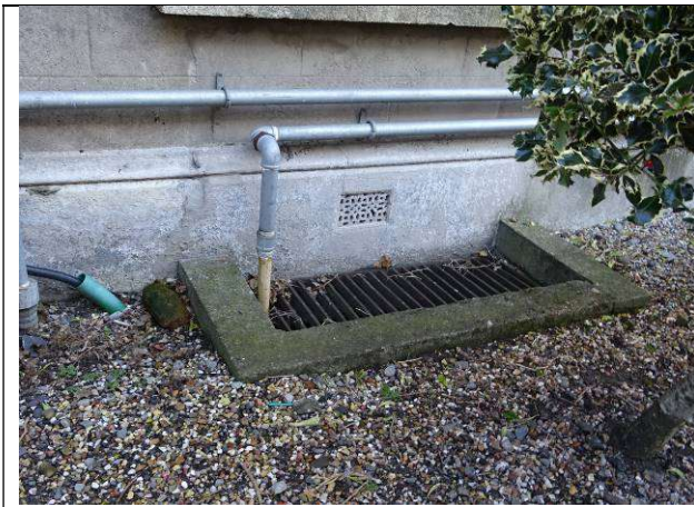
Fig.77: Iron grille to basement lightwell
