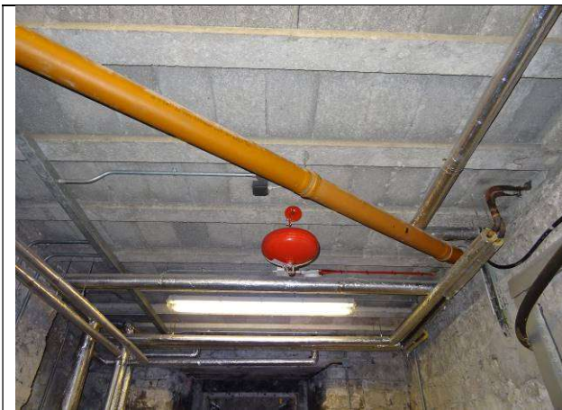
Fig.91: Precast concrete joists and slabs to ceiling
