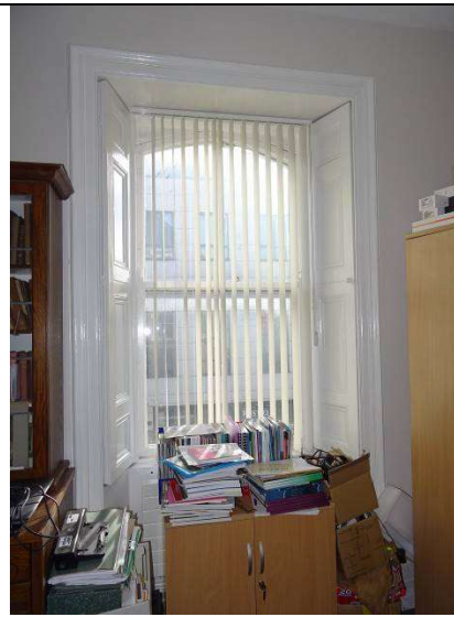
Fig.168: Window on south elevation
