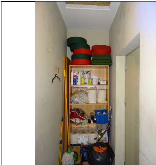
Fig.125: Store to north of children's reading room
