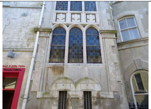
Fig.86: First floor of stairs bay to west
