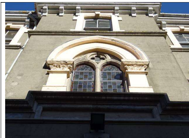
Fig.75: First floor of entrance bay
