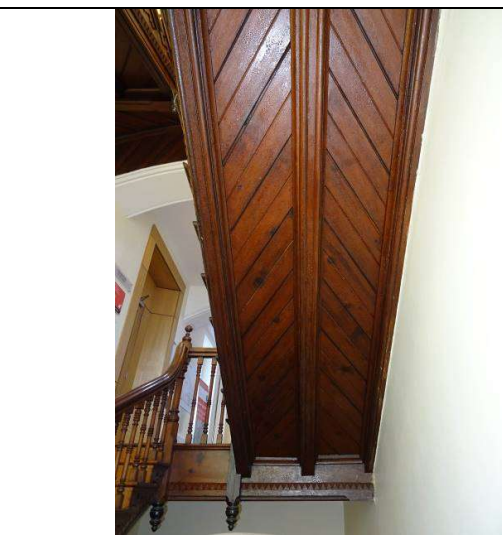
Fig.146: Underside of second flight
