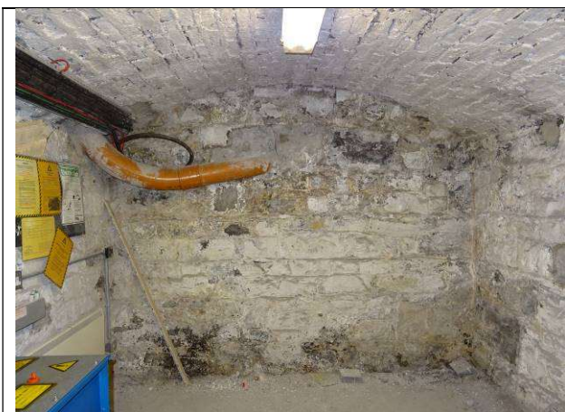
Fig.93: Basement, mid room, looking south
