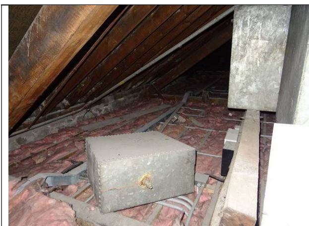
Fig.199: Insulation between ceiling joists to east end of roof
