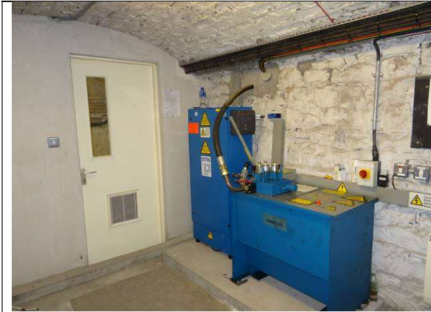
Fig.95: Basement, mid room, looking northeast
