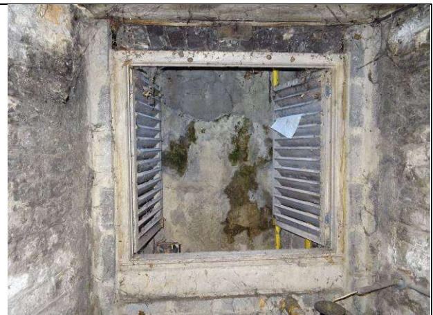
Fig.92: Basement, east room, south window ope
