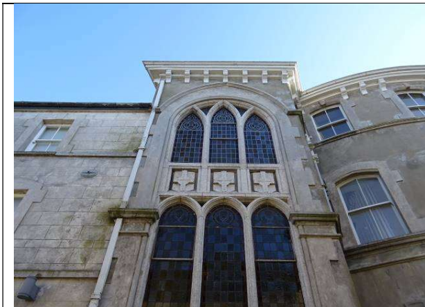
Fig.85: Second floor of stairs bay to west
