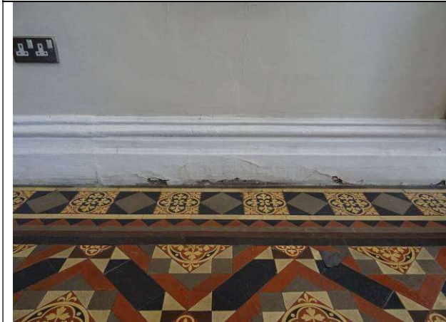
Fig.107: Entrance hall, skirting boards and encaustic tiles
