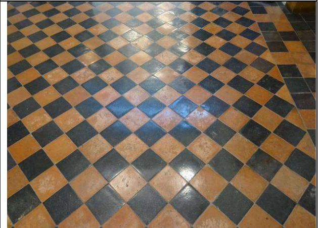
Fig.108: Black and red terracotta quarry tiles to stairhall
