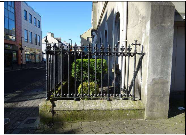
Fig.78: Iron railings and granite plinth to front
