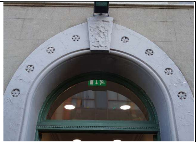
Fig.72: Decorative surround to entrance door
