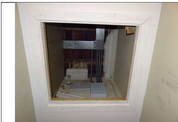
Fig.127: Original ceiling laths with run-in-situ cornice above suspended ceiling
