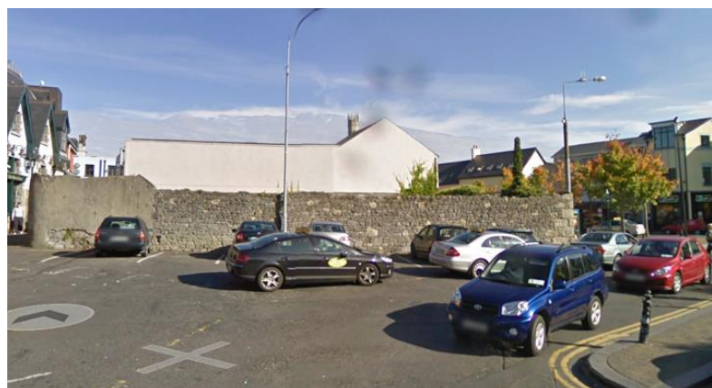
Pic 2: Existing elevation from the Southerly carpark side
