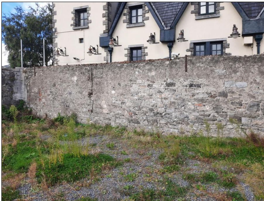
Pl. 7 Close-up View of West Boundary.
