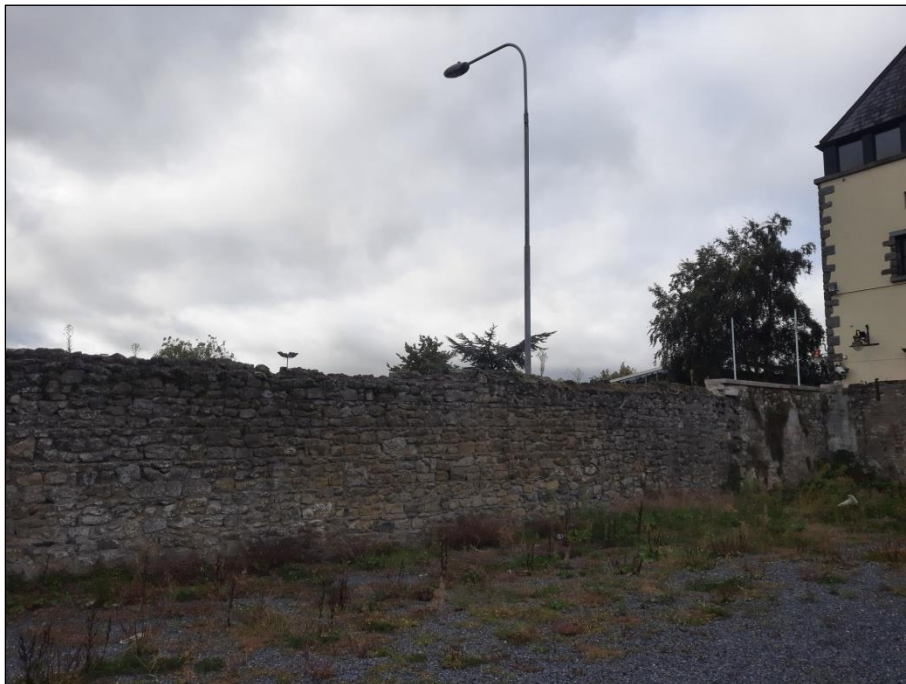
Pl. 5 South Boundary Wall.
