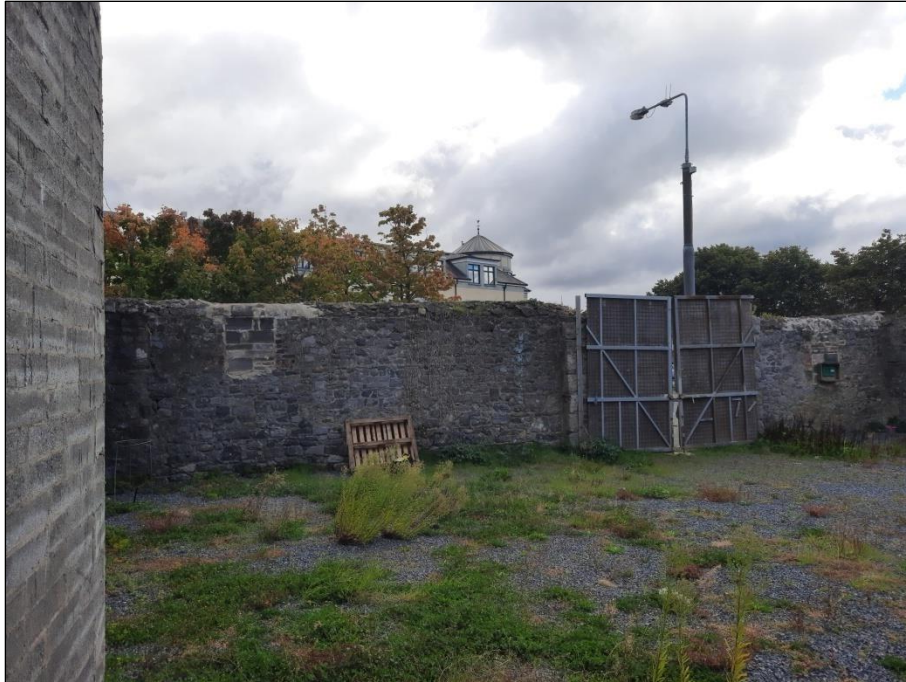
Pl. 8 East Boundary Wall with Gated Entrance.
