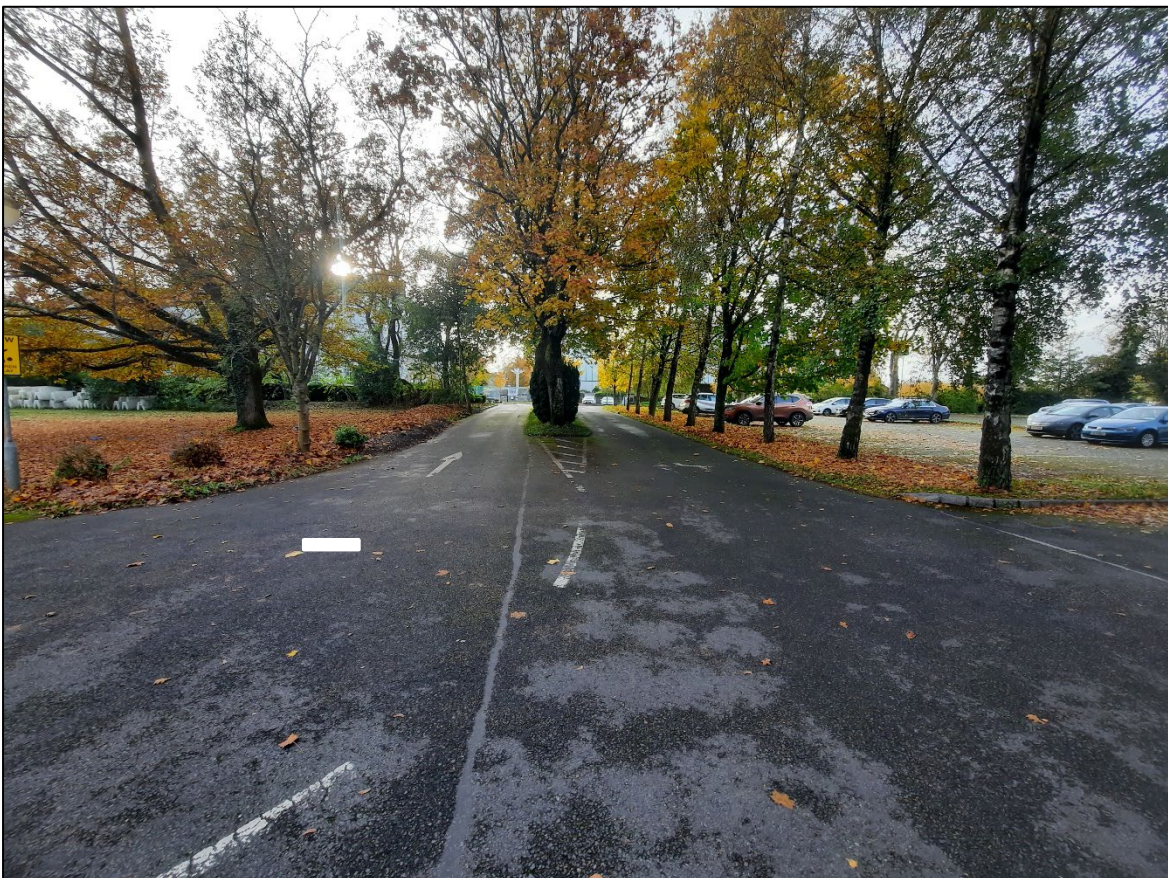
Photo 2: View from beside Lennon Hall looking west towards Visual along the vehicular entry exit route.
