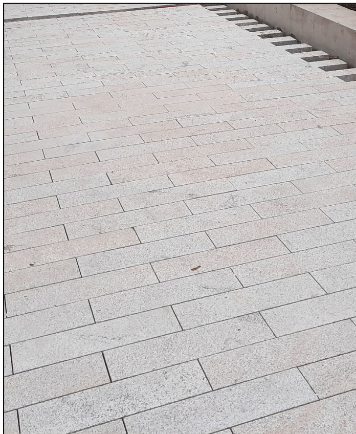
Photo 5: Proposed paving type(Tan / Grey Granite with Dark Grey Granite or Blue / Grey Limestone features) or similar approved. Source Stonepave
