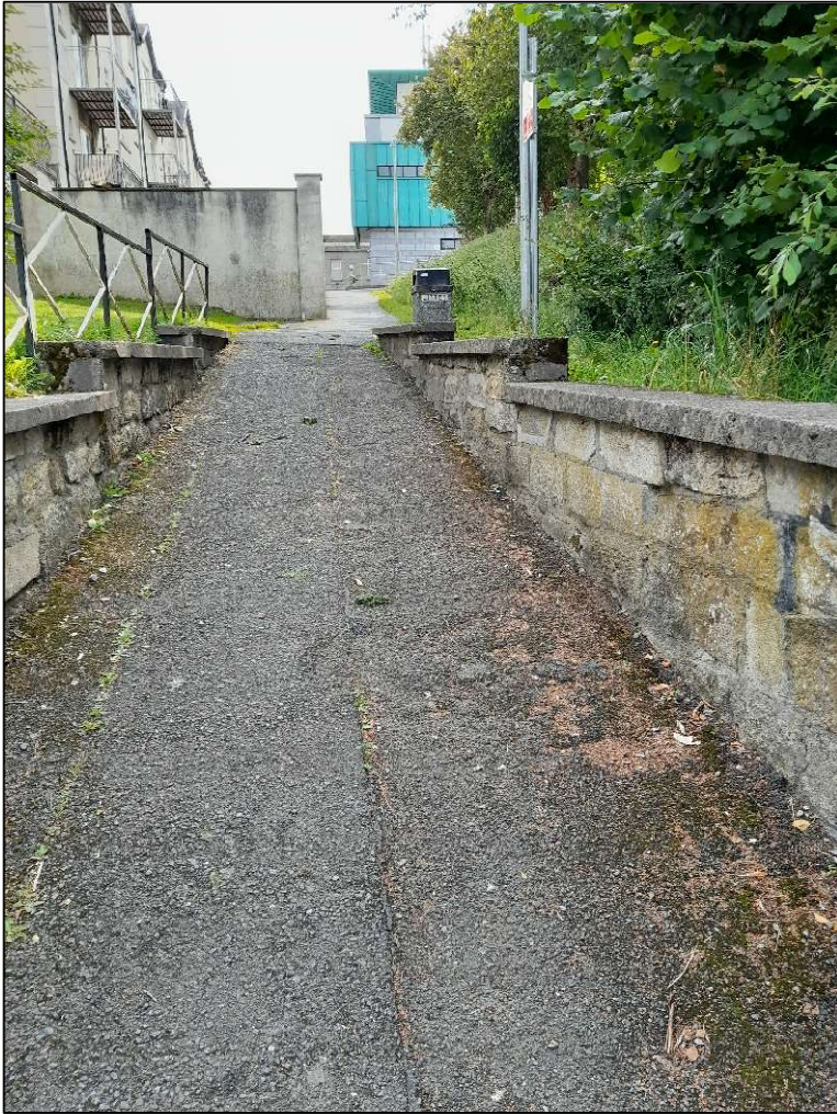
Photo 3: View looking south along existing ramp towards Market Square
