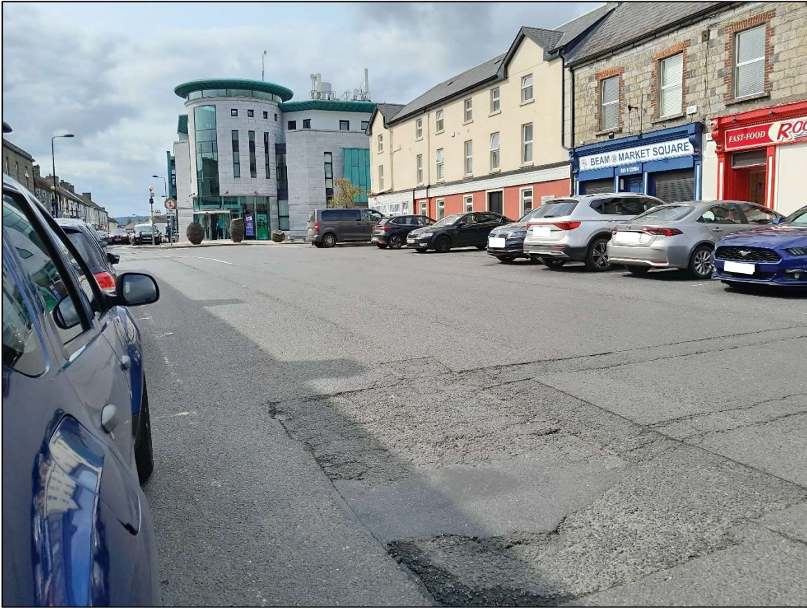
Photo 1: View looking west along Market Square to the Credit Union
