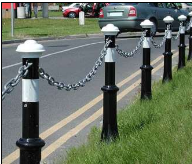
Photo 13: Proposed bollard and chain type or similar approved to be fitted at the top of the embankment (Source IPL Group)
