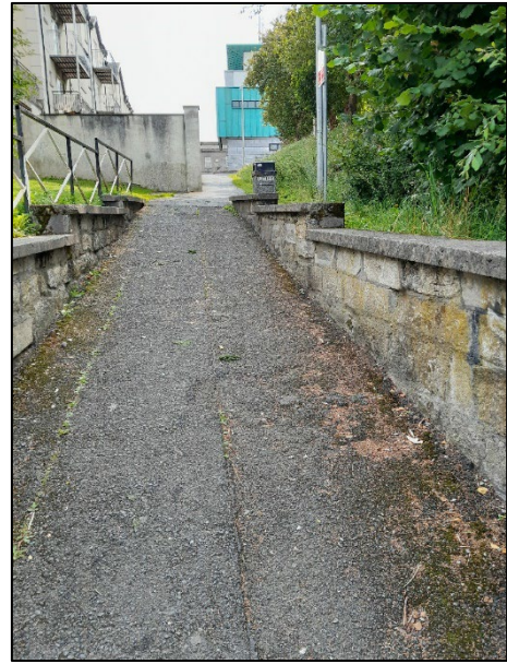
Fig. 07 - Looking south along existing ramp.
