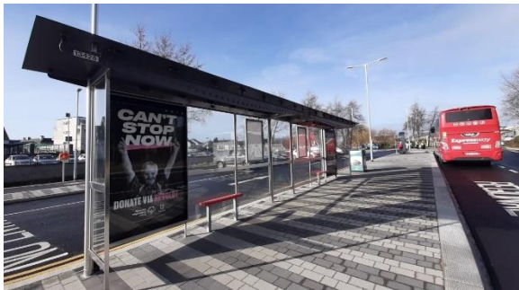
Carlow Bus Park Upgrade
