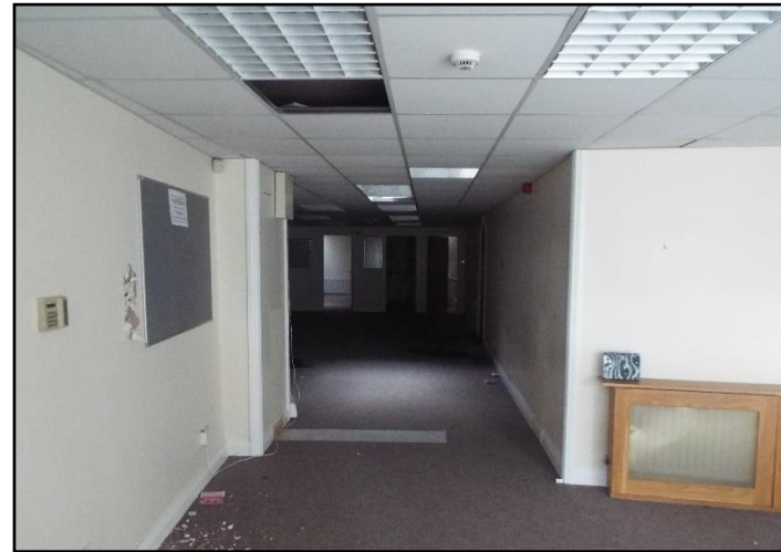
Plate 4: Building No. 16 inside (BL3)
