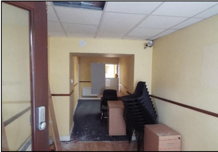
Plate 5: Building No. 15 inside (BL3)
