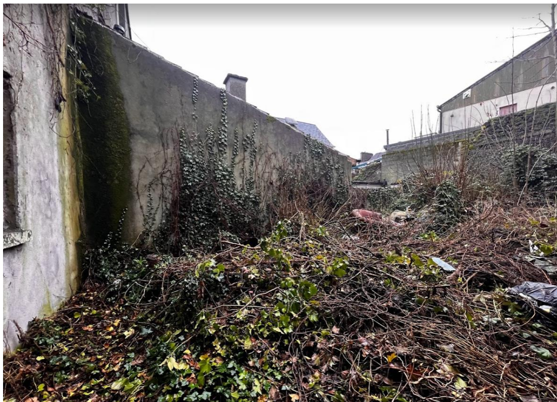
Plate 4: Western boundary wall at No. 1 Haymarket.
