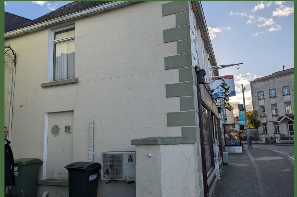
Fig 1.11 View looking West
