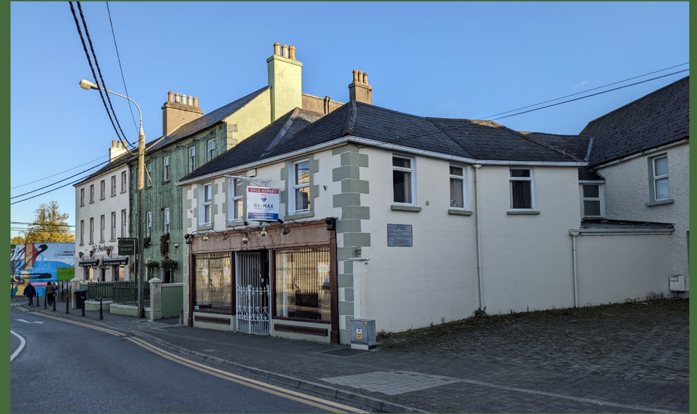
Fig. 1.9 View looking East
