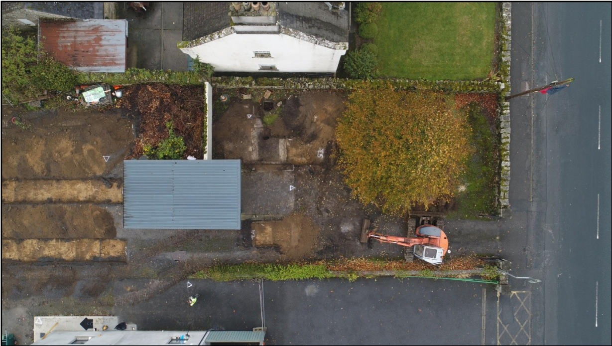
Plate 12 - Vertical drone image of the proposed development site showing location of underground structure relative to Borris Garda Station on the adjoining property (01.11.2019).
