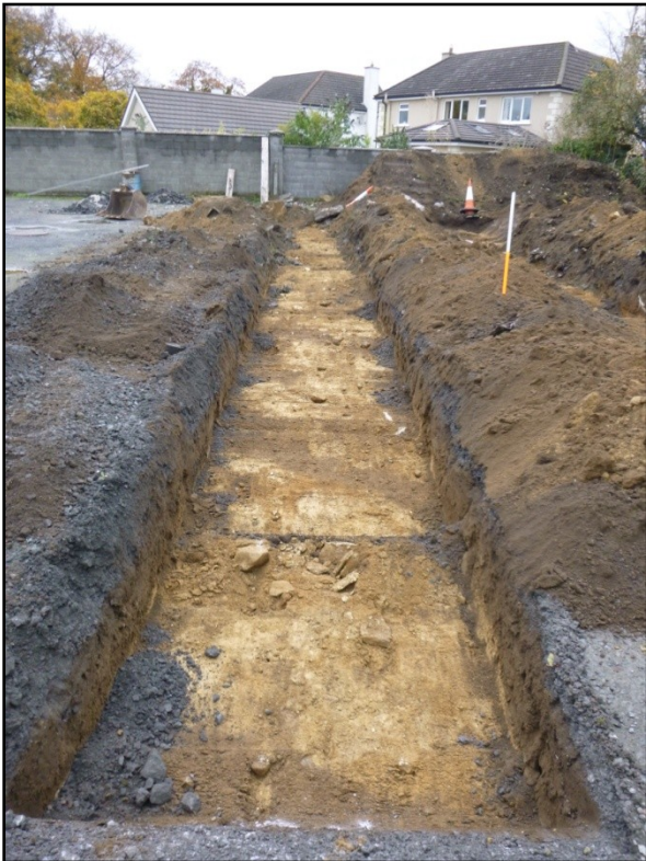
Plate 6 - Test trench 3 from S-N (01.11.2019).
