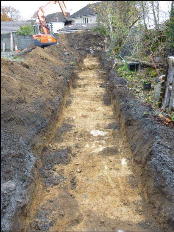
Plate 3 - Test trench 1 from S-N (01.11.2019).
