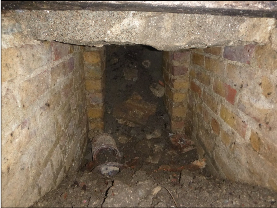
Plate 11 - Underground cell/passage as viewed E-W from box opening (02.09.2019).
