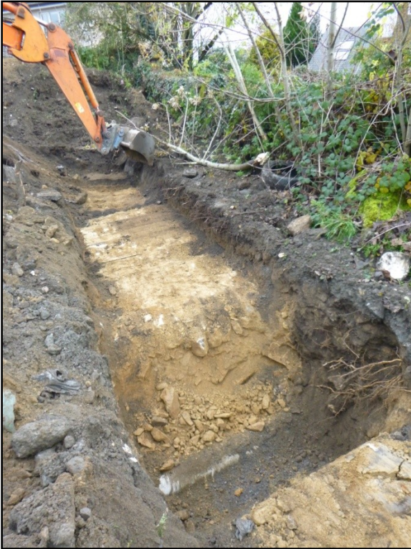
Plate 4 - Concrete storm water pipe in Test trench 1 (01.11.2019).
