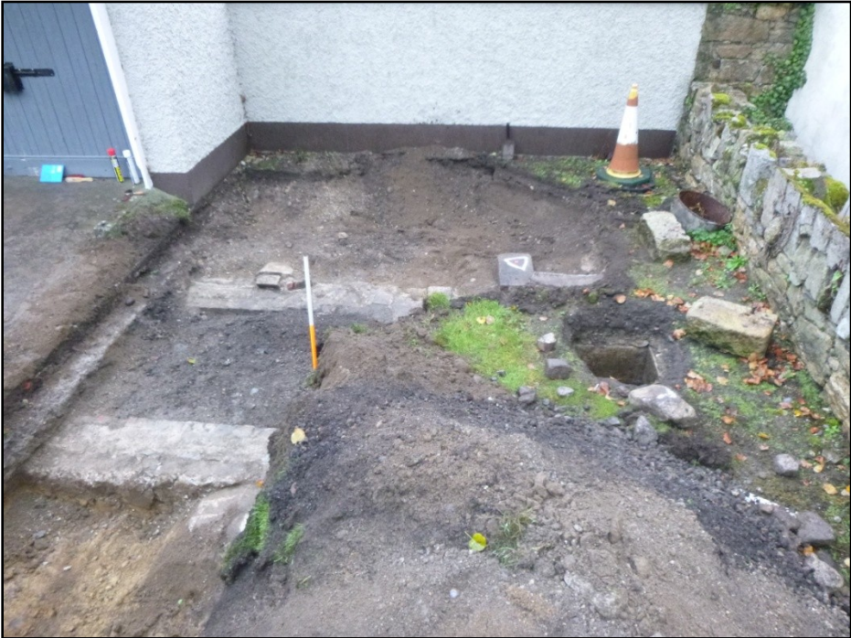
Plate 10 - Test trench 5 from S-N across underground cell/passage structure (01.11.2019).
