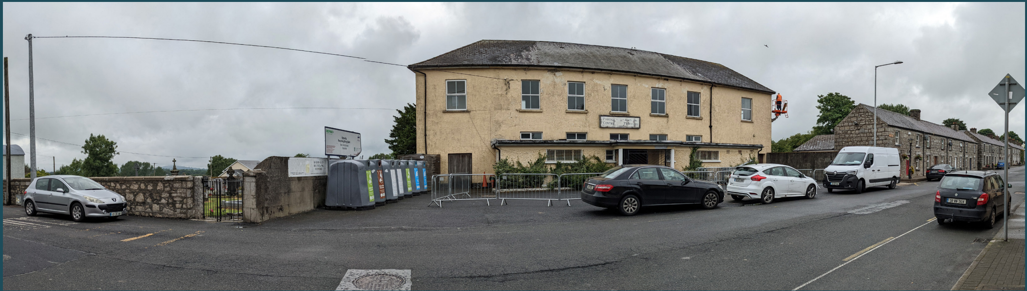
Fig. 1.4 Existing Site Panoramic View - Showing original 5 Bay Schoolhouse building Center with later additions to the front and sides
