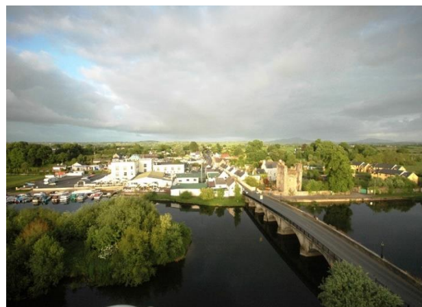
Aerial view of Leighlinbridge looking west across the River Barrow.
