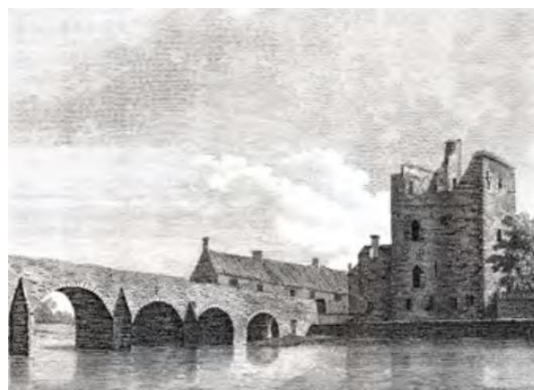
LEIGHLIN BRIDGE, S.W. ASPECT, 1840/50
