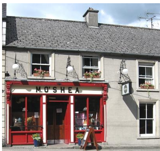
Figure 12.11: Traditional Shopfront in Borris
