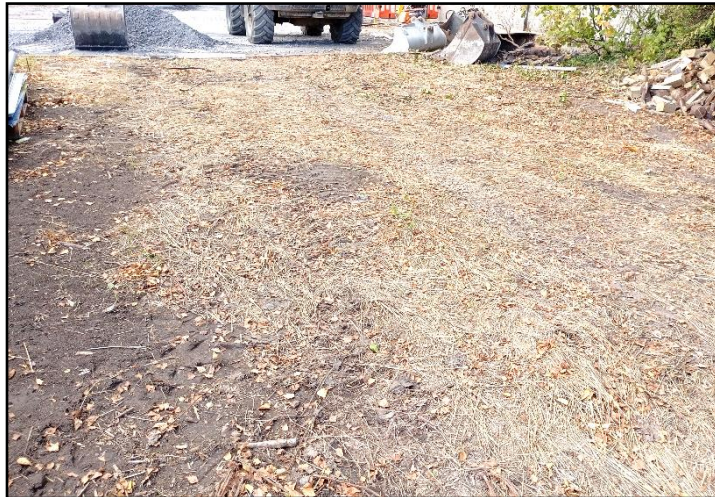
Plate 3: Spoil and bare ground (ED2)
