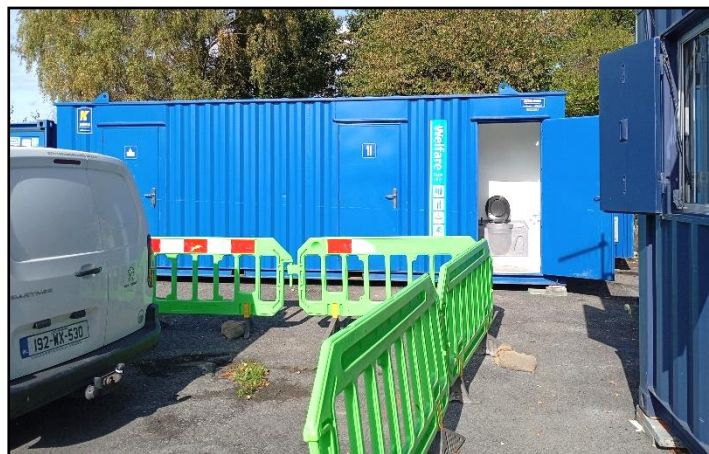
Plate 8: Temporary offices (BL3)
