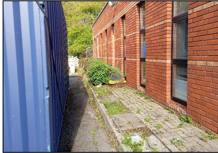
Plate 2: Rear of the existing building (BL3)
