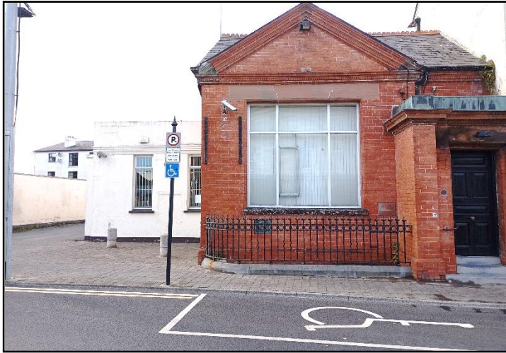
Plate 1: Site entrance (BL3)
