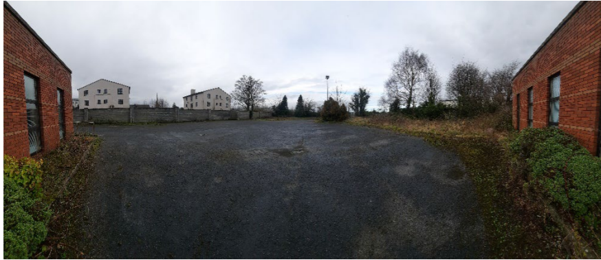
Photo 03 : View from the end of the building looking towards the western shared boundary, a private site, towards the river.
