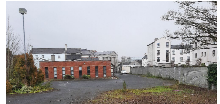
Photo 02: View from the rear of the site looking at the shared boundary with the adjoining apartment scheme.
