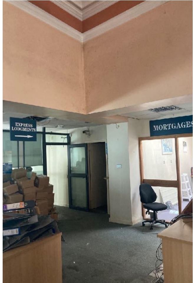
Rear corners of banking hall where original walls have been removed and beams inserted. It is proposed to reinstate the partitions/walls in this space to reinstate the original enclosure
