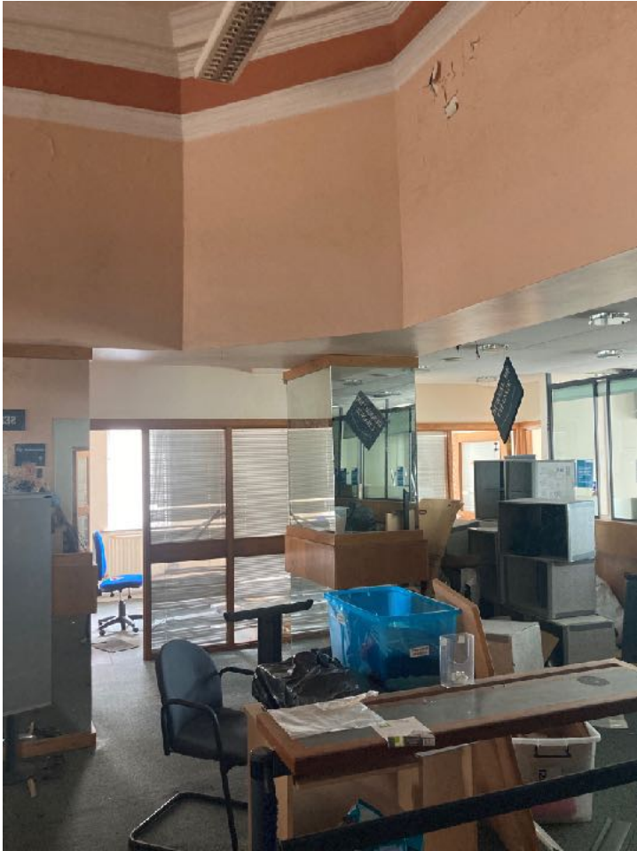
Rear corners of banking hall where original walls have been removed and beams inserted. It is proposed to reinstate the partitions/walls in this space to reinstate the original enclosure
