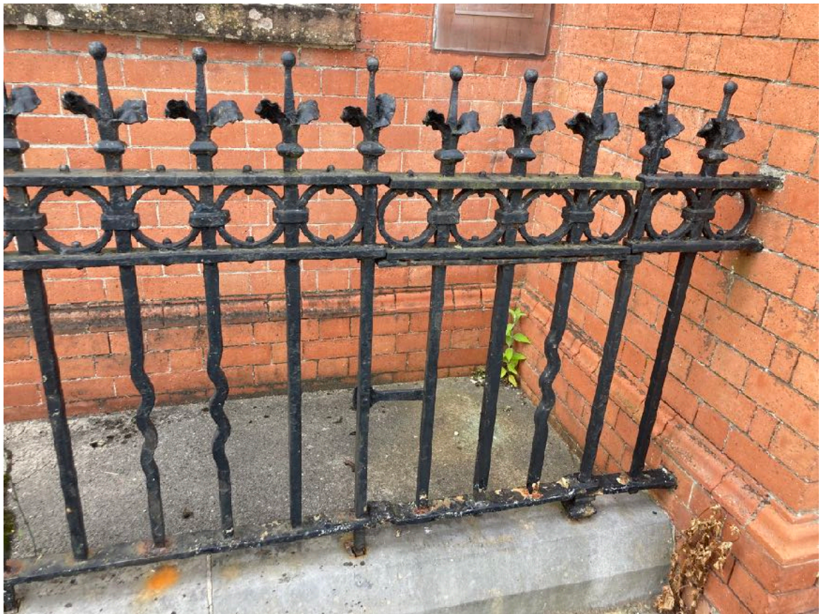
Front railings to banking hall - probably wrought and cast iron
