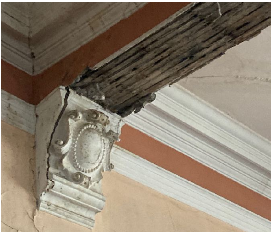
Rear corners of banking hall where original walls have been removed and beams inserted. It is proposed to reinstate the partitions/walls in this space to reinstate the original enclosure
