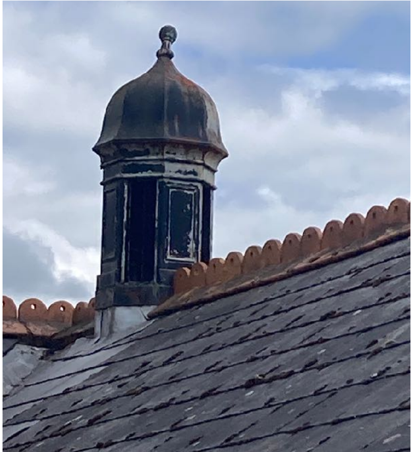
Octagonal ventilator feature on roof, to be retained
