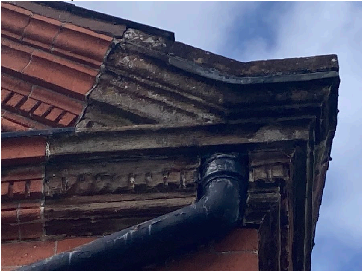
Eaves pieces (granite or reconstituted stone) formed to match profile of brick barge
