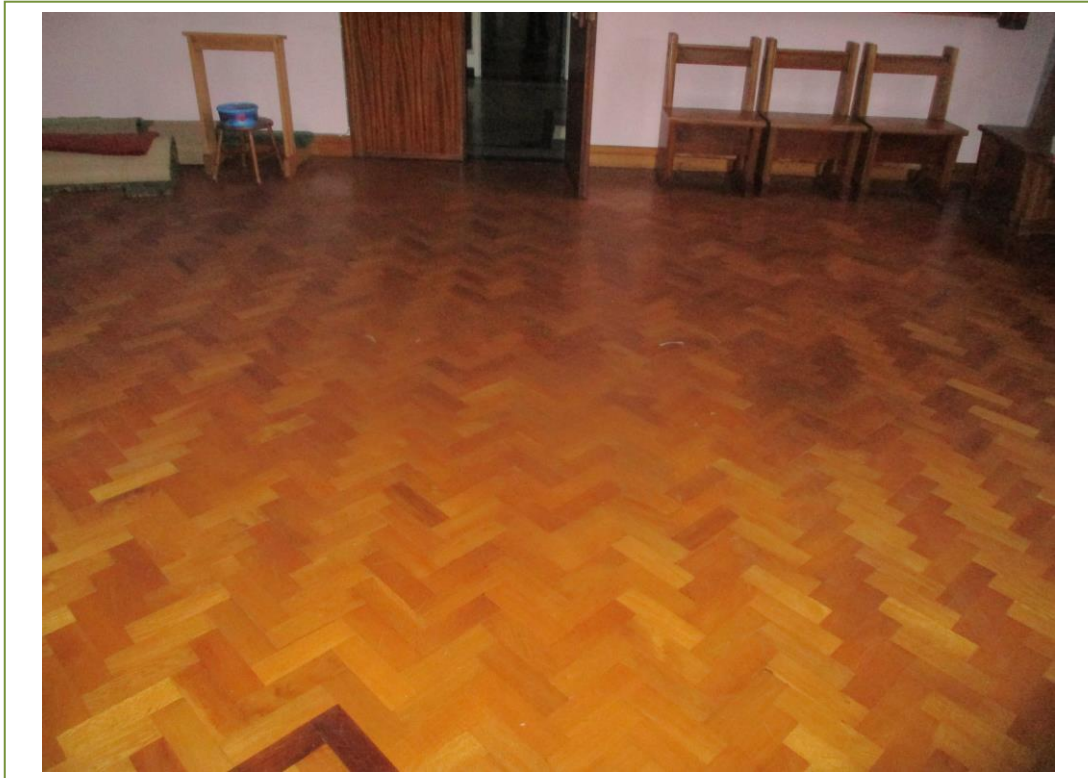
Original Timber floors
