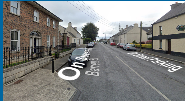
Fig 2.5 On Street Parking -North end of Barrett Street looking South
