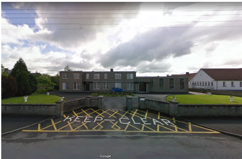
Fig. 2 – Existing entrance from Long Range showing stone clad boundary wall
