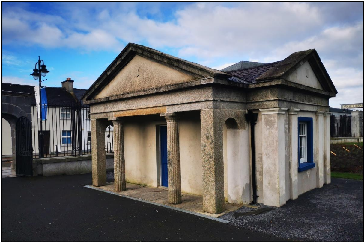
Figure 5.1: Building at Carlow College entrance along the L4025 – low bat roost potential – to stay
