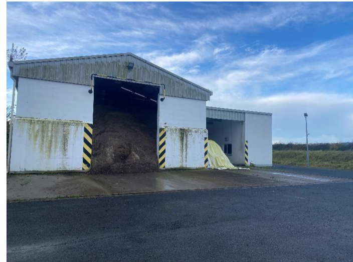
Plate 5.4: Viewpoint No. 3.1 – Macadam yard looking south-west
