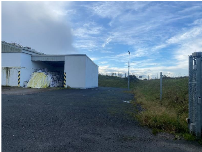
Plate 5.3: Viewpoint No. 2.2 – Site entrance looking south
