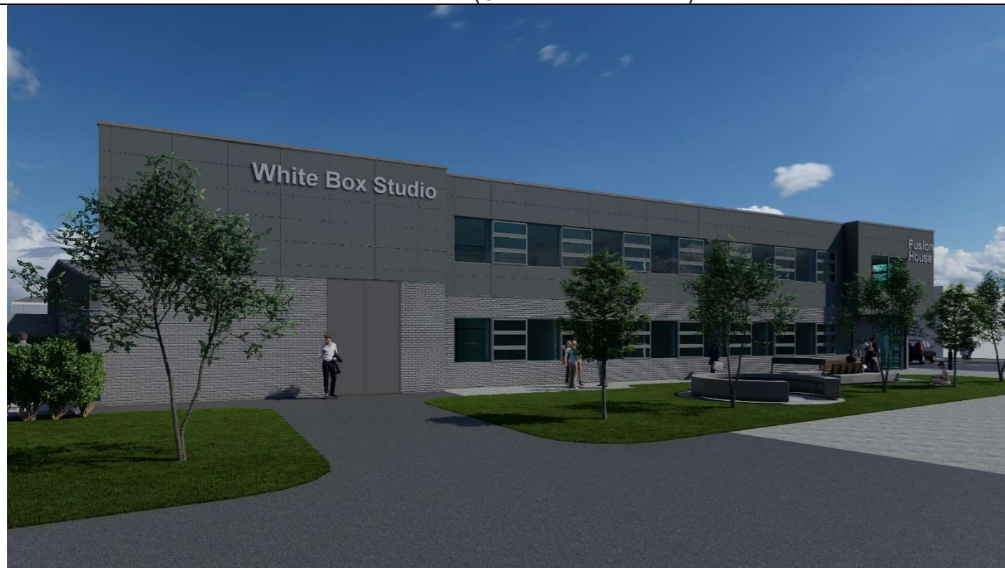
2 Fusion House (Office Accommodation)
