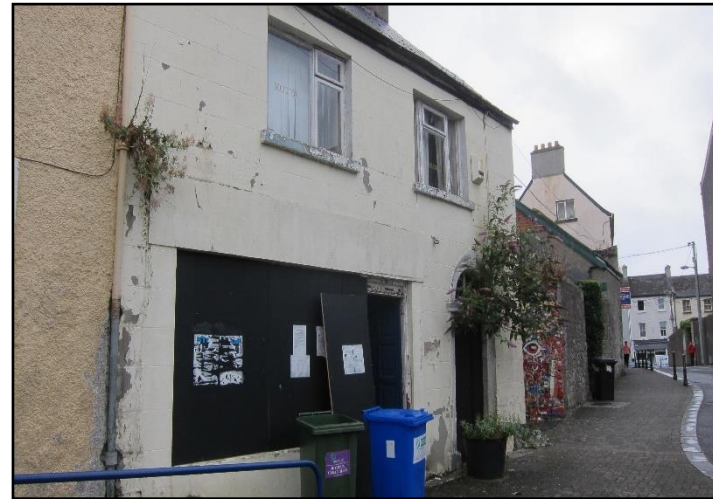
Plate 4: View of site along road boundary
