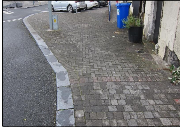
Plate 6: Footpath along front of building
